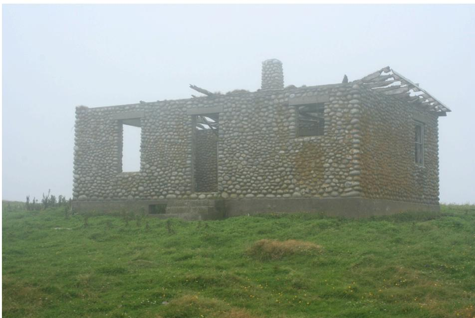
Figure 3 - As of July 2014, the beach stone building erected in 1949 remains on Outer Bald Tusket Island, although the roof has become detached as the result of a recent hurricane (author's photograph, 2014).
