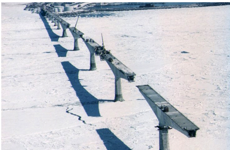
Figure 3 - The Confederation Bridge, under construction (Baird.com)
