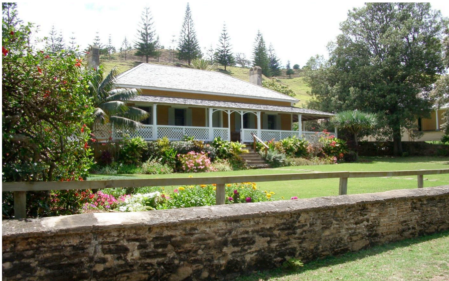
Figure 4 - A Heritage Building along Quality Row, Kingston (photograph by the author)
